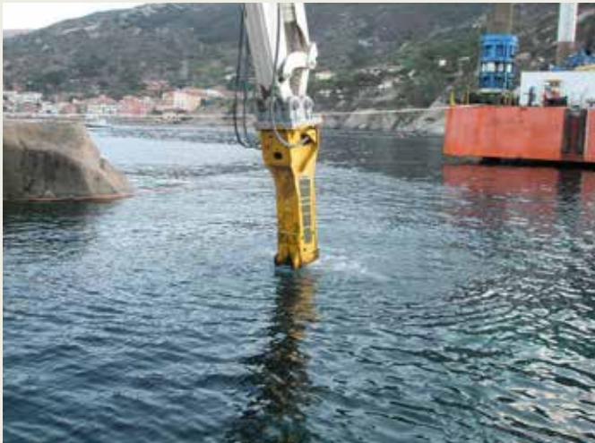
HB 4100 underwater rock excavation in Italy
