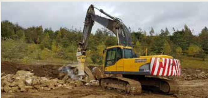
HB 2000 on the 30t excavator reducing sandstone (Yorkstone) boulders on the dedicated area for the secondary breaking
