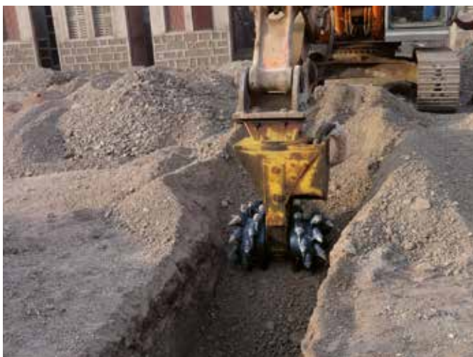
Transverse drum cutter ER excavating trenches
