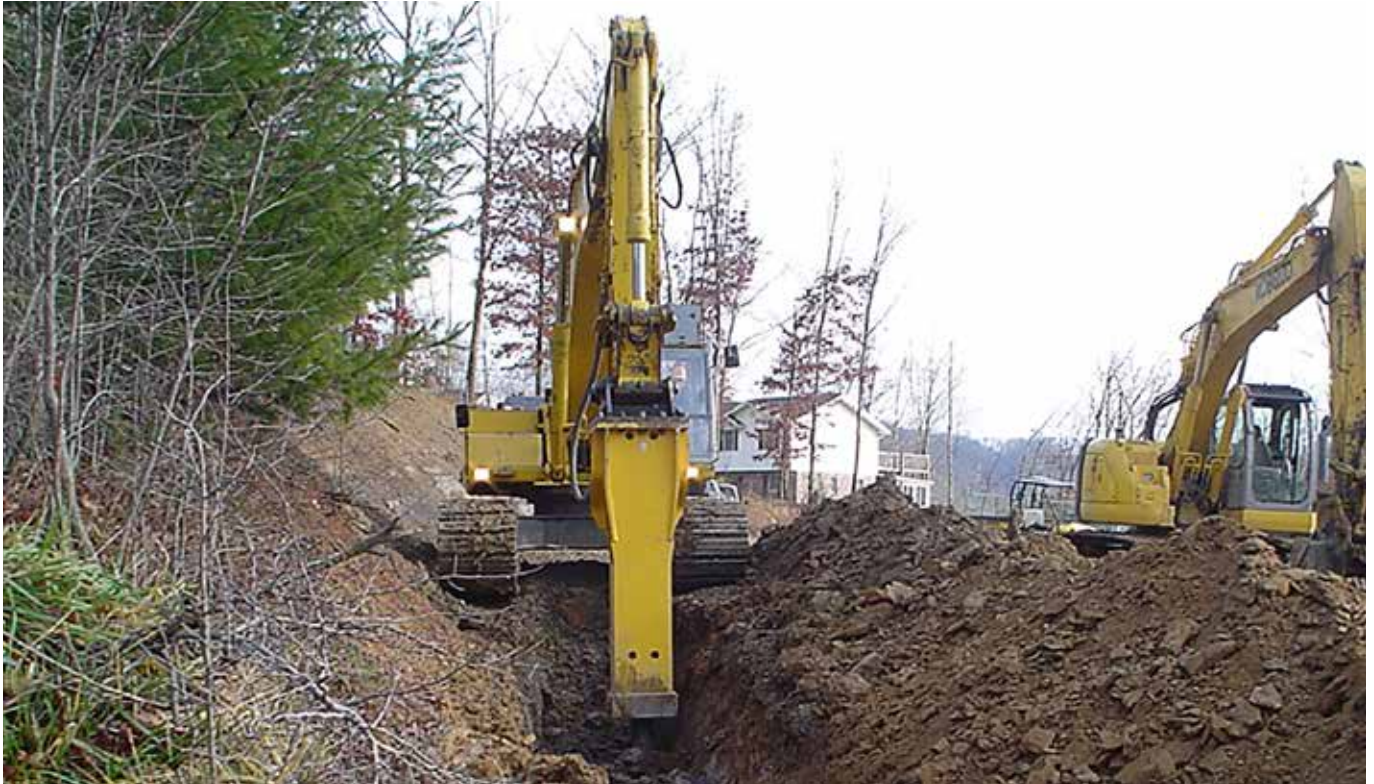
Trenching with hydraulic breaker
