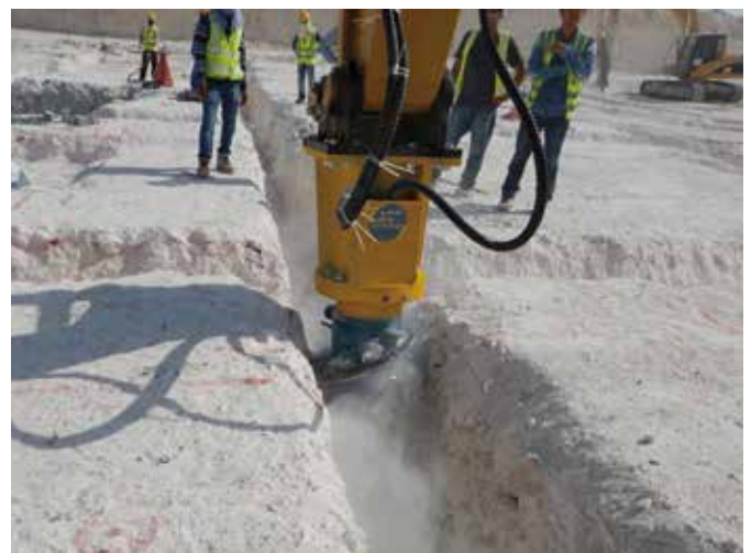
Axial Drum Cutter ER-L excavating trenches for foundation
